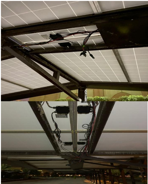
inverters, DC combiner, AC combiner, and the value of produce DC
